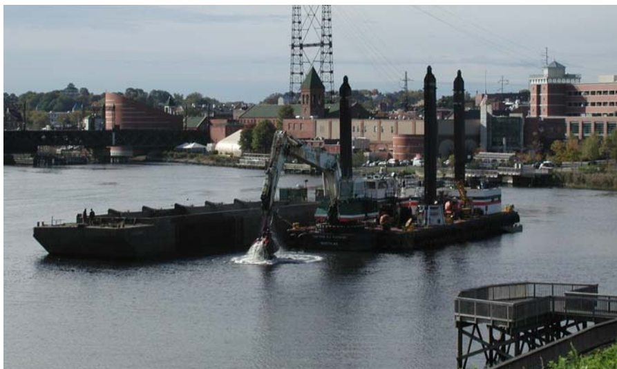
View of the dredging from Phase 1; Photo by Tony Mobilia
